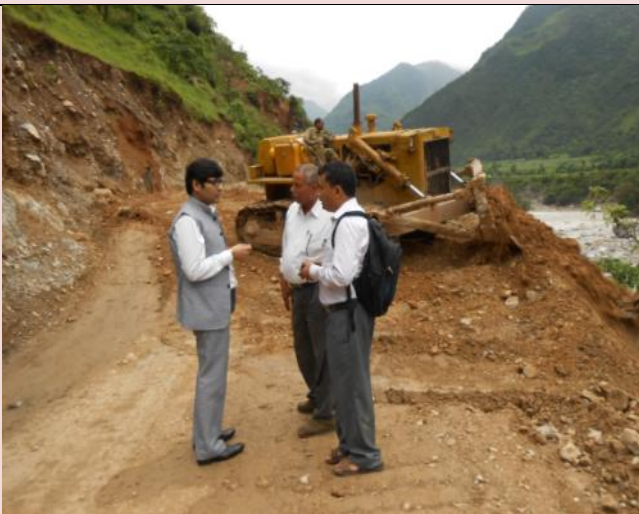
Road being re-established
